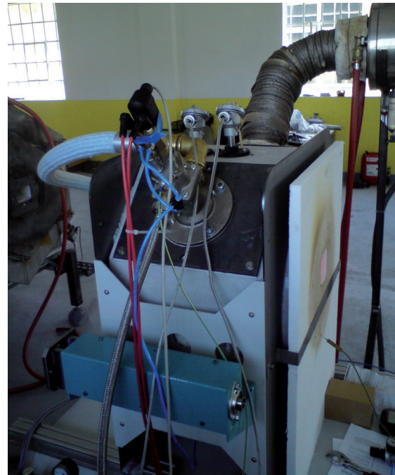
fig.: Installation of hebö prototype oven
